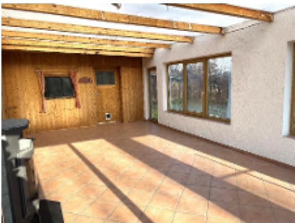
...in die Garage
